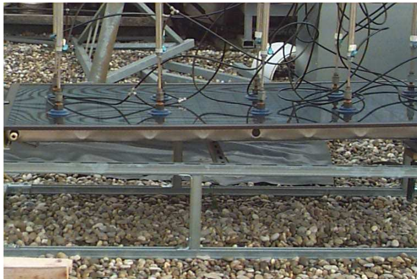
Figure 3: Positive pressure test of the collector cover
